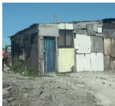
A TYPICAL INFORMAL HOUSE IN SWEET HOMES, KHAYELITSHA
