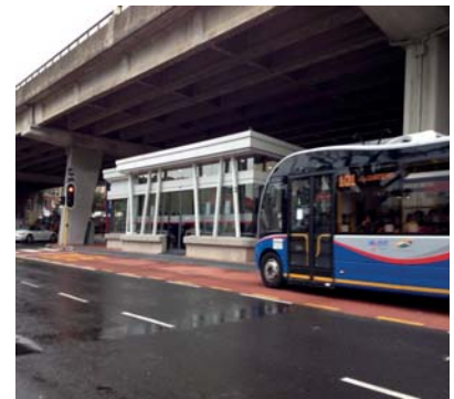
MYCITI BUS AND FEEDER STATION, GARDENS
